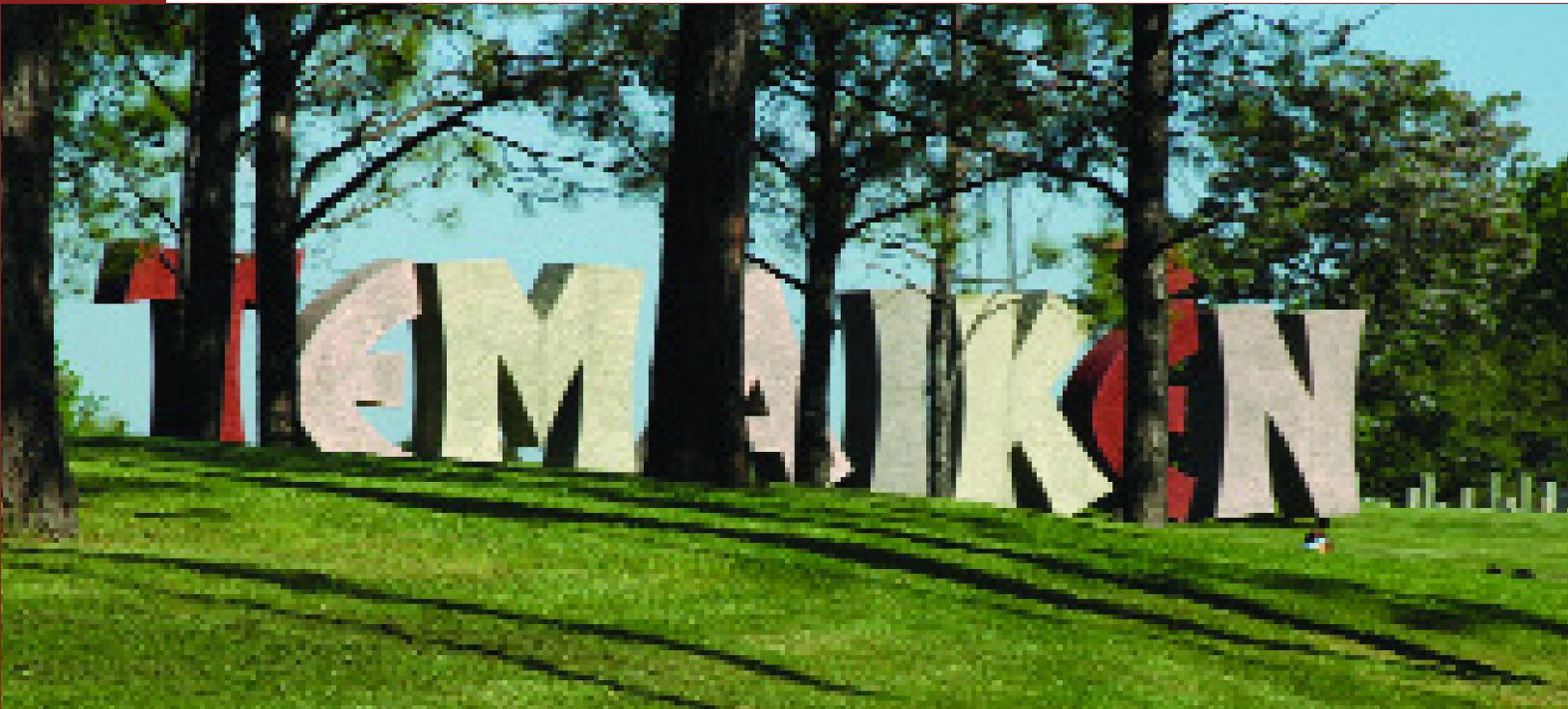
The 8-by-65-ft. Temaikèn Zoo entrance sign is a steel structure with metallic mesh and projected-concrete letters, set on a concrete foundation. The colors reflect the zoo's emphasis on earth and nature.
